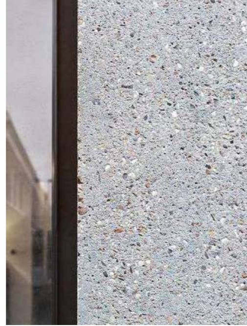
Washed concrete walls with burnished aluminium window frames
